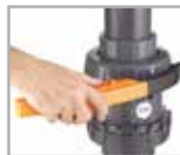
Nuts tightening
